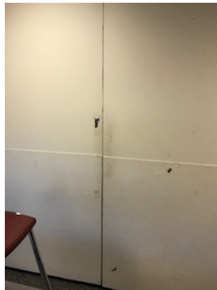
Dividing walls failing with noise bleed between classes
