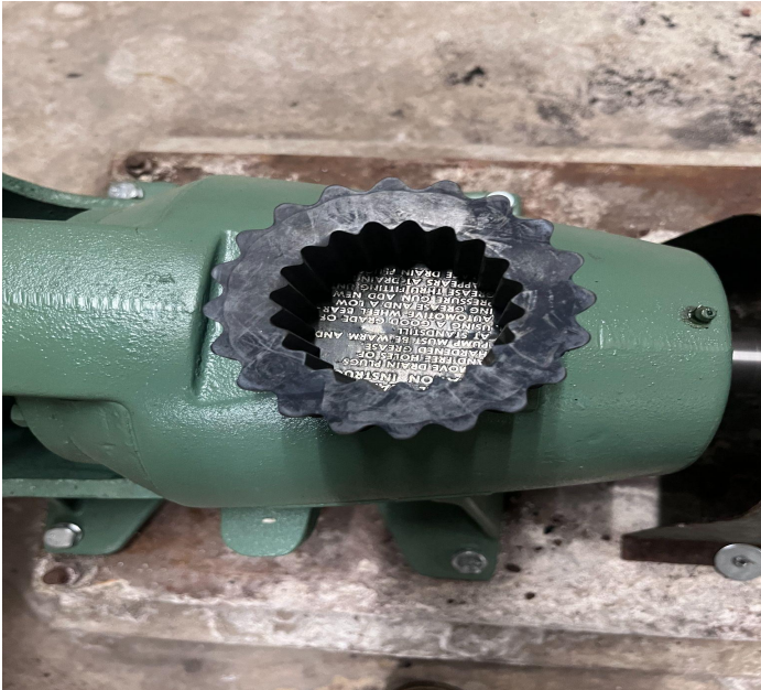
Replaced coupler on hot water pump #2
