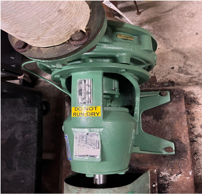
Boiler pump #1 rebuild
