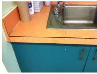
Figure 12 - Plastic Laminate counter delaminating.
