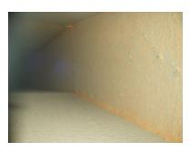
Figure 3 - Interior of Ductboard showing build-up of dust.
