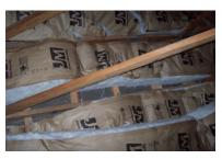
Figure 6 - Picture taken before renovations showing R=19 attic insulation not properly installed.
