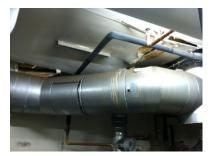
Figure 9 - Boiler room ceiling has breaches in the fire rating.
