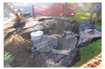
Figure 4 - Drywell during construction in 2005.
