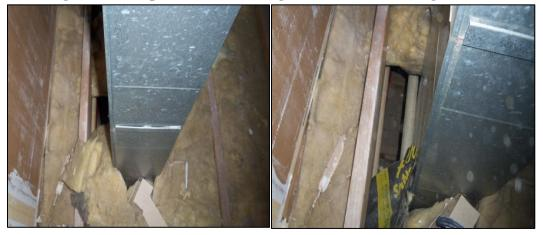
Image 7 depicts the result of an improperly sealed air barrier and underperforming thermal barrier. The electrical chases extend through the acoustic tile ceiling, puncture through the air barrier with fiberglass batting plugging the hole against leakage.
