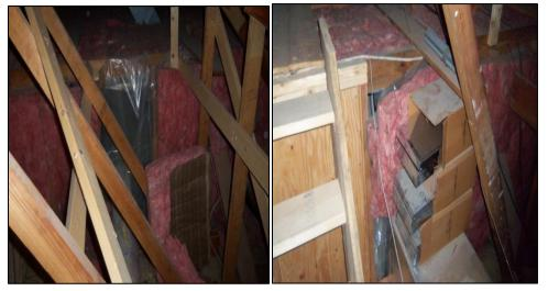
The insulation in image 5 has been installed to manufacturer's specifications. Fully lofted no gaps or compression points and fully encapsulated with an air barrier. Image 6 depicts the challenges in maintaining a continuous sealed air barrier and high performing fiberglass insulation. The best management practice for the HVAC penetration would involve sealing around the metal duct work – where ever the air barrier exists – and reinstalling insulation around the duct work.
