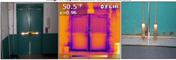
Image 1: Typical exterior door construction
