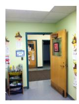
Figure 10 - Door with built-in door stop prevents closer from operating.
