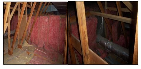
Image 3: Attic knee walls with poorly sealed HVAC penetrations
