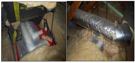
Image 9: A fair air barrier (with limited penetrations) and thermal barrier over duct work
