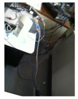
Figure 8 - Power strips plugged into power strips are against fire code.
