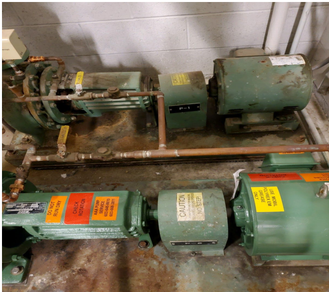
Hot water pump 1 leak repair
