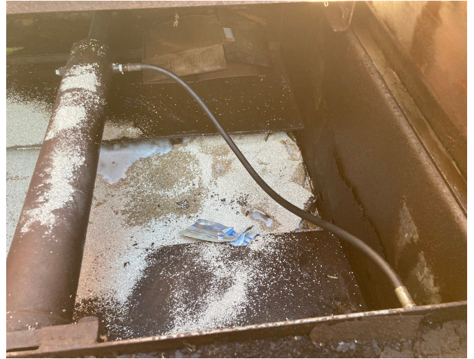
Annex trash compactor hydraulic repair
