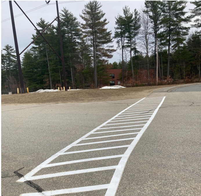
Crosswalk line striping
