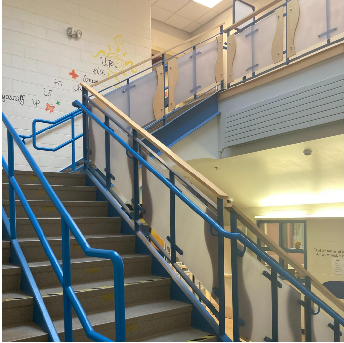
Annex stairwell painted railings
