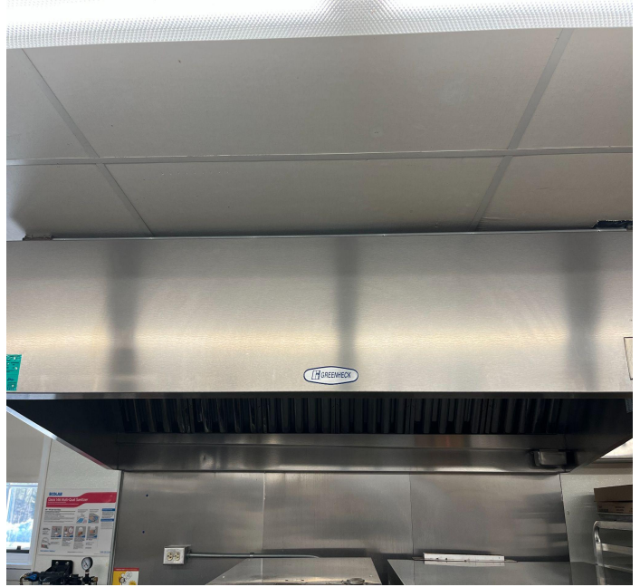
Kitchen hood inspection
