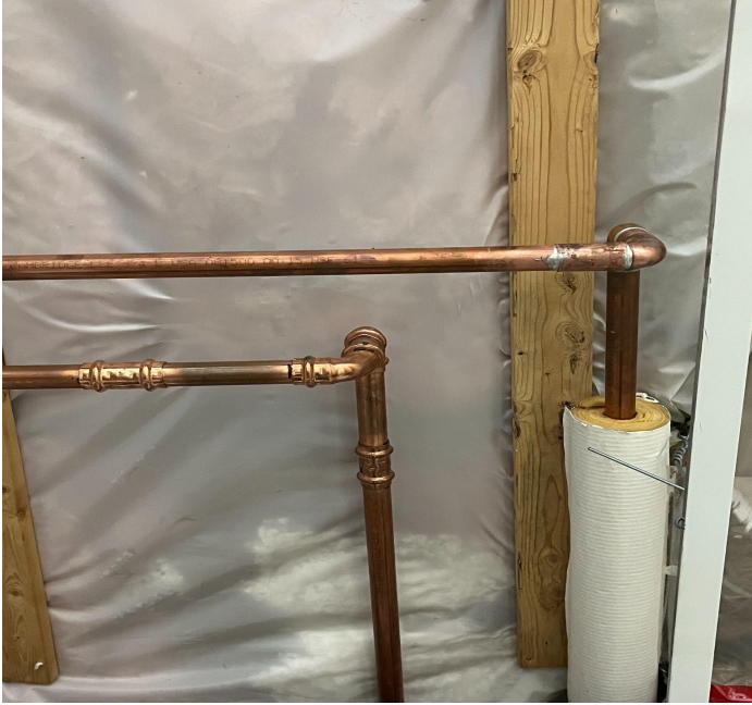
Replaced broken plumbing piping in kindergarten room
