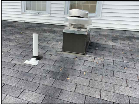
P4: REMOVE, STORE AND REINSTALL ALL CURB WRAPS. PROVIDE NEW WRAPS AROUND CURBS WHERE WRAPS ARE NOT CURRENTLY INSTALLED.
