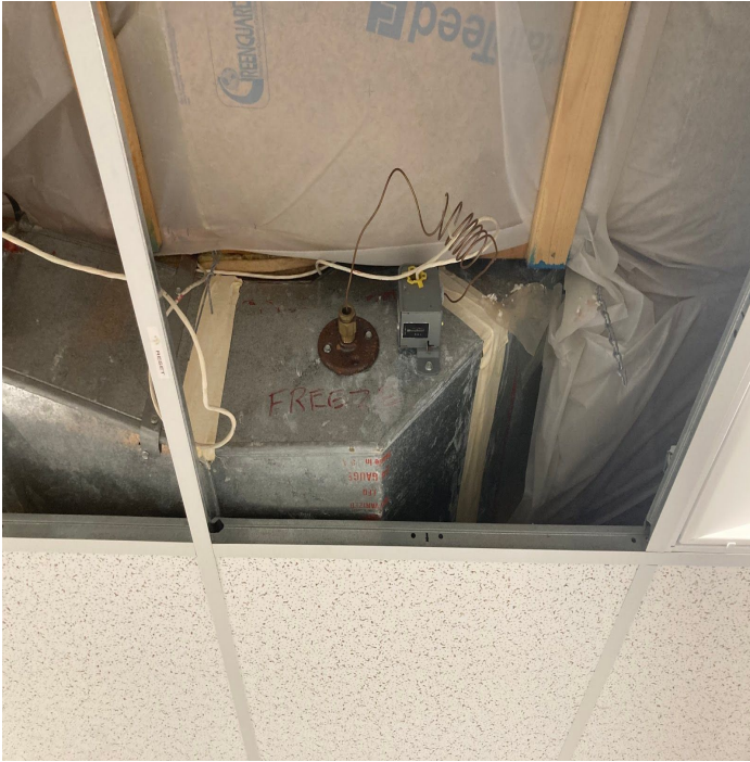
Tripped freeze stat (W8), boiler #1 fuel piping, new energy management system, new vacuum
