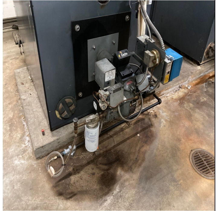
Tripped freeze stat (W8), boiler #1 fuel piping, new energy management system, new vacuum
