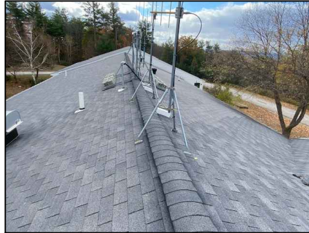
P5: REMOVE STORE AND REINSTALL THE BALLAST SYSTEM. PROVIDE NEW 12"x12" SLEEPER "PADS" UNDER ALL SUPPORTS FASTENED TO THE ROOF AREA.
