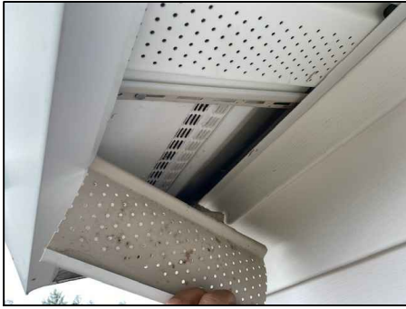
P1: REMOVE BOTH SOFFIT LEVELS PER THE PLANS AND SPECIFICATIONS.
