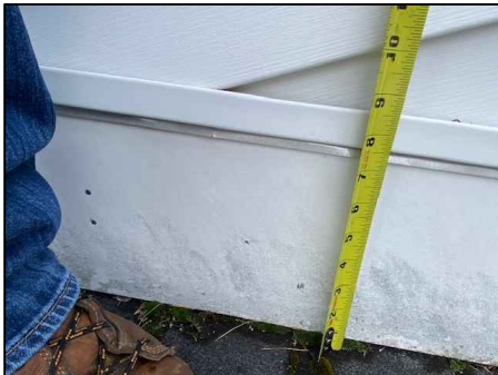
P7: REMOVE, STORE AND REINSTALL THE EXISTING TRIM BOARDS. REMOVE ALL NAILS AND OTHER FASTENERS. REUTILIZE THE SAME HOLES WITH FASTEN MASTER CORTEX TRIM SCREWS AND COLOR MATCH PLUGS.
