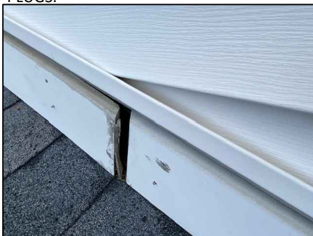
P10: THE TRIM SHALL BE REINSTALLED WITH OVERLAPPING SCARF CUTS AND MATERIAL COMPATIBLE GLUES.
