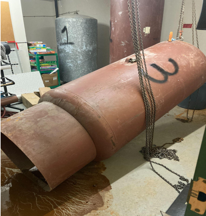
Domestic water tank bladder replacement
