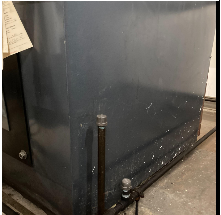
Fuel piping risers removed
