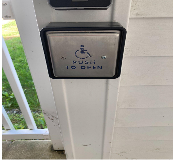
ADA access button repair
