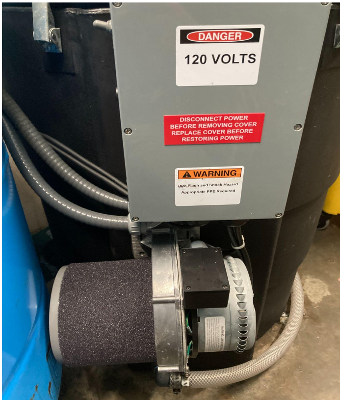
Clearadon motor replacement
