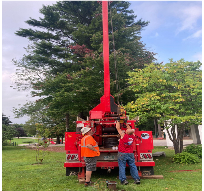
Removing well pump
