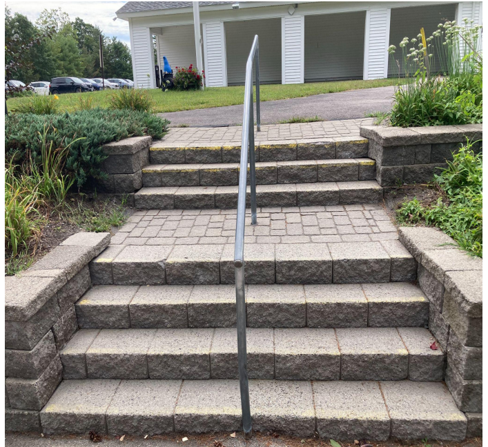
Wall and stair repair/rebuild
