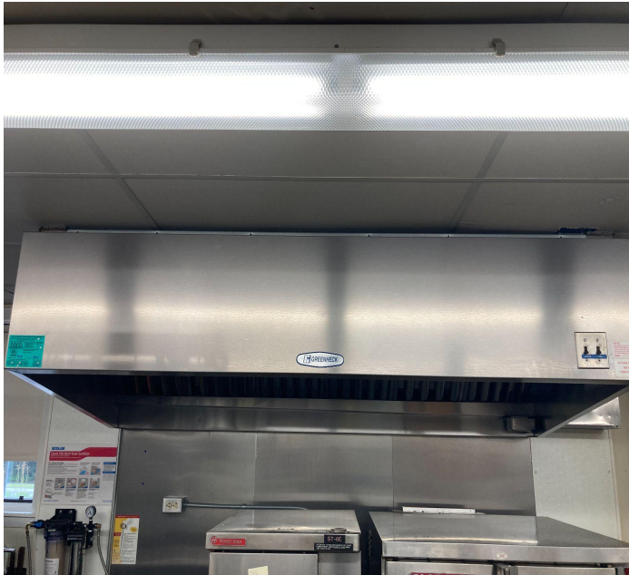
Kitchen hood inspection
