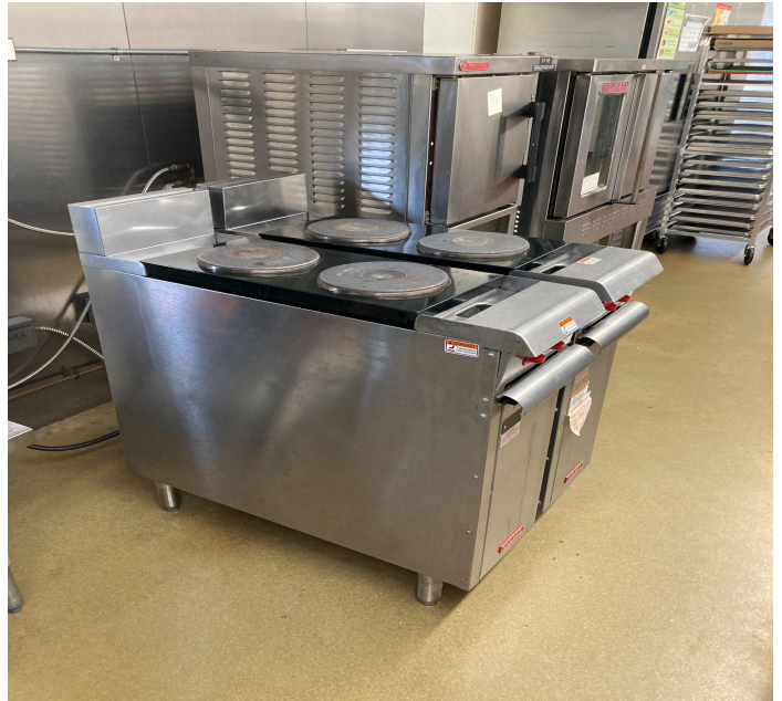
Kitchen hood oven shutdown
