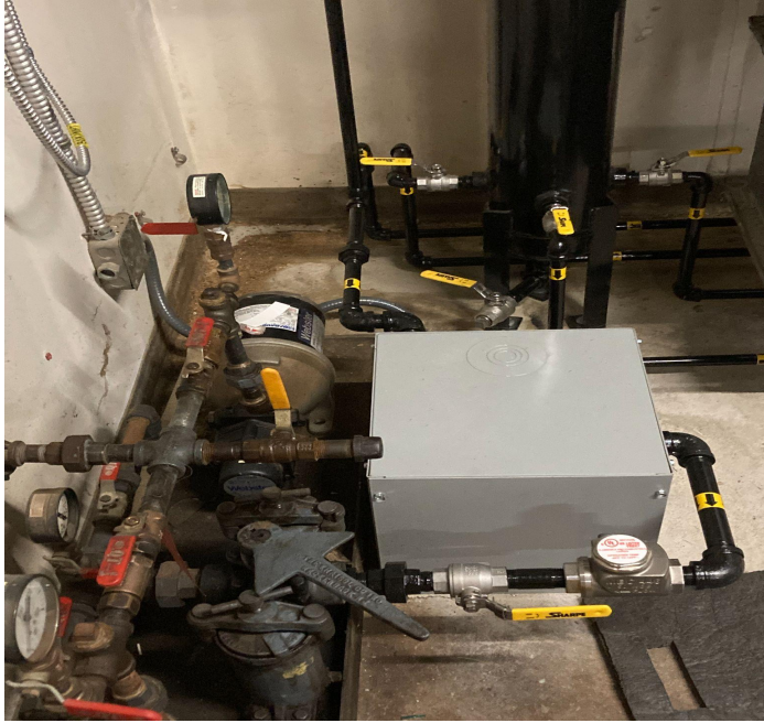
Underground storage tank piping repair
