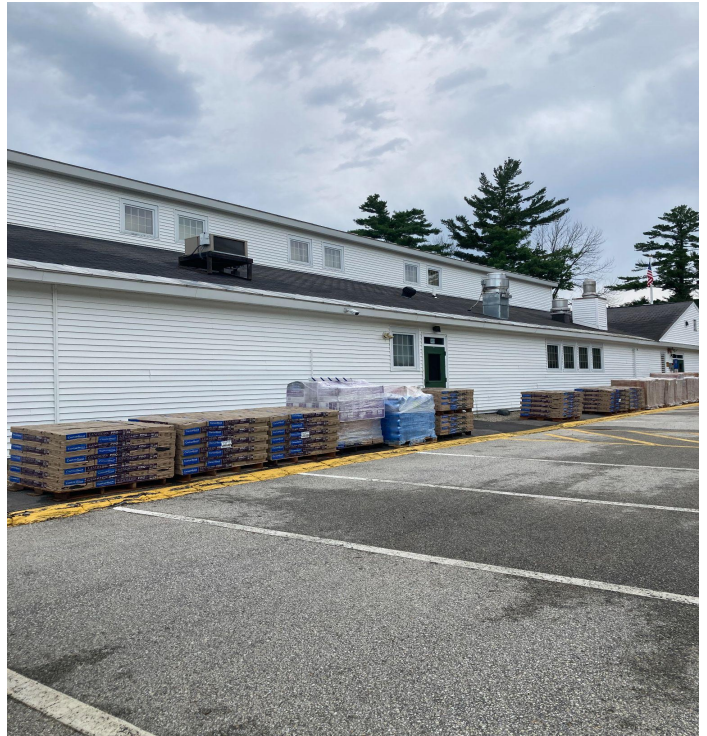
Roof material delivery
