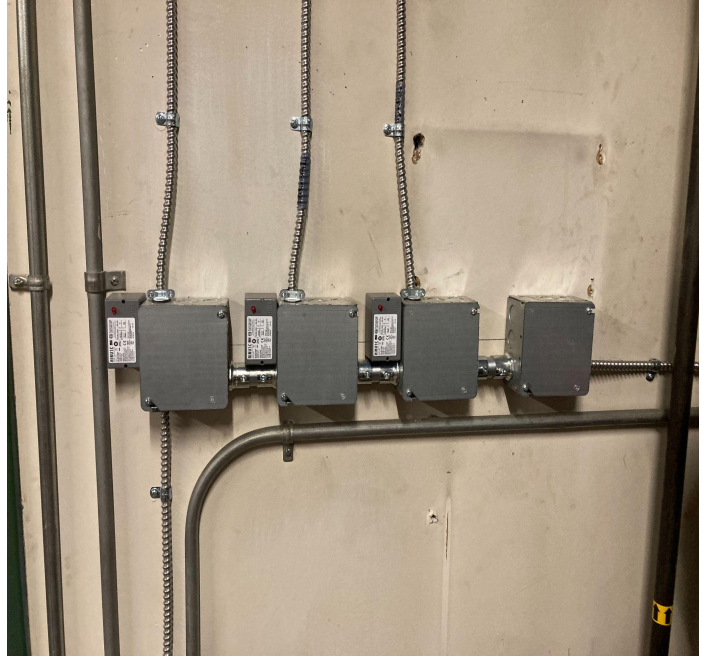
Underground storage tank electrical repair
