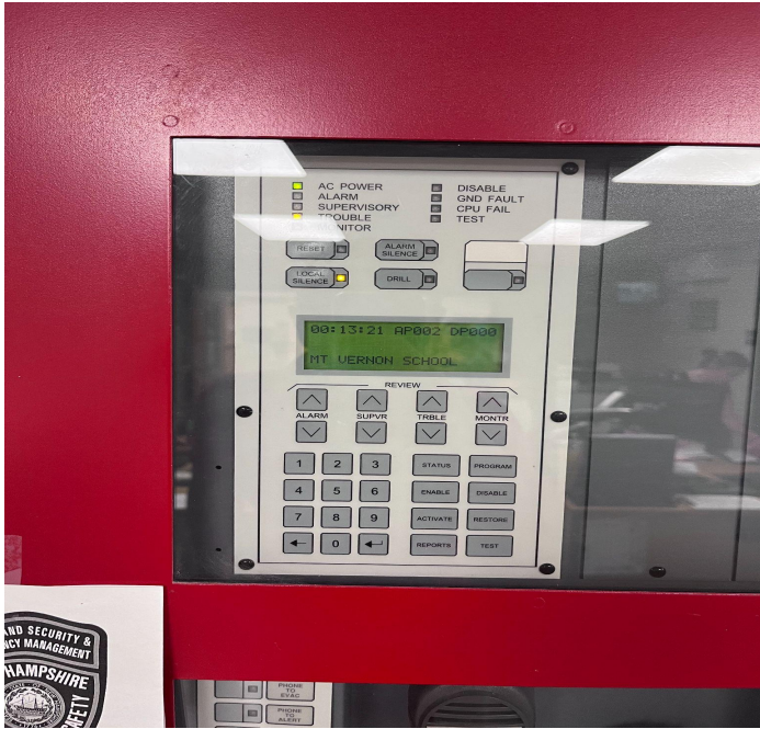
Fire panel trouble call for device mapping error
