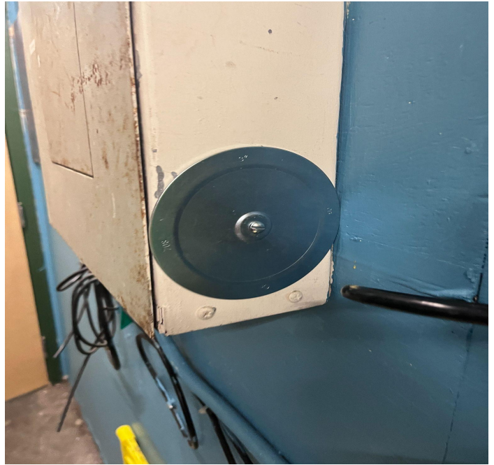
Installed knock out seal in water room electric panel
