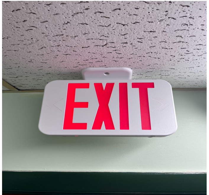
Emergency exit light inspection and repair
