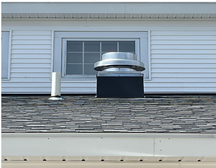
Replaced damaged exhaust fan on roof
