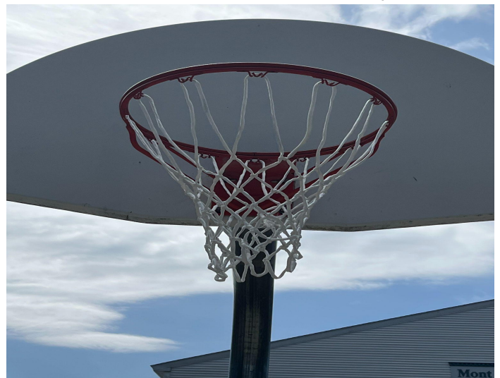
Installed new nets for outdoor hoops
