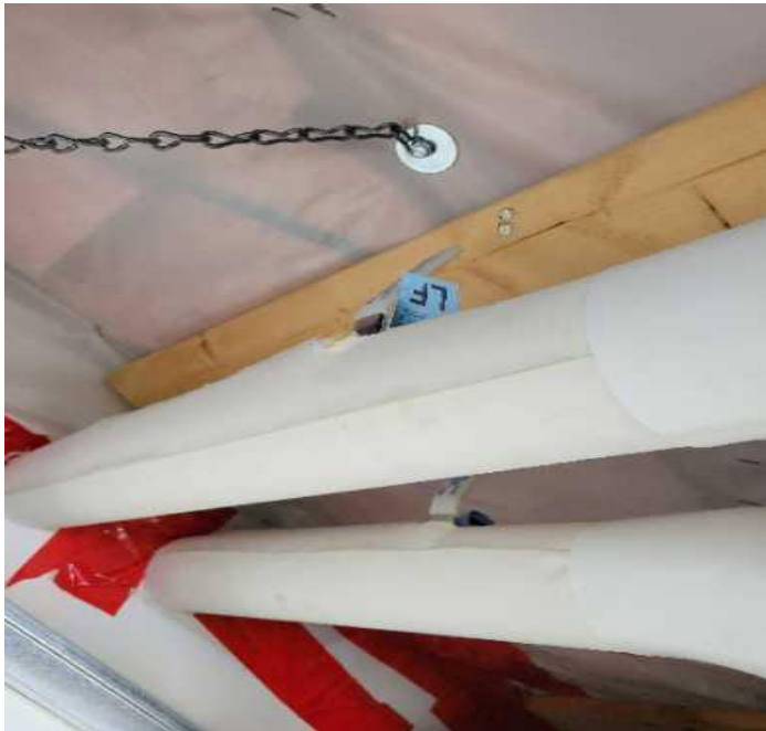
Installed shut off valves for kindergarten room plumbing
