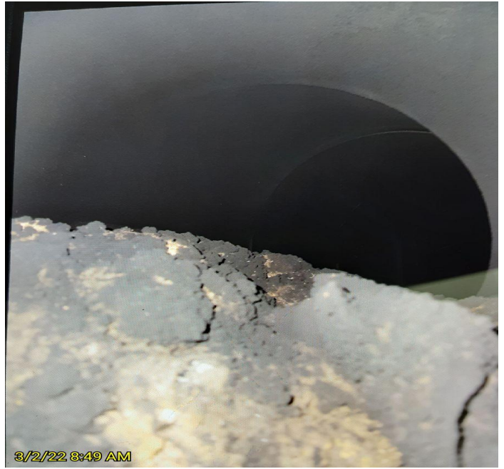
Boiler breeching PCB testing
