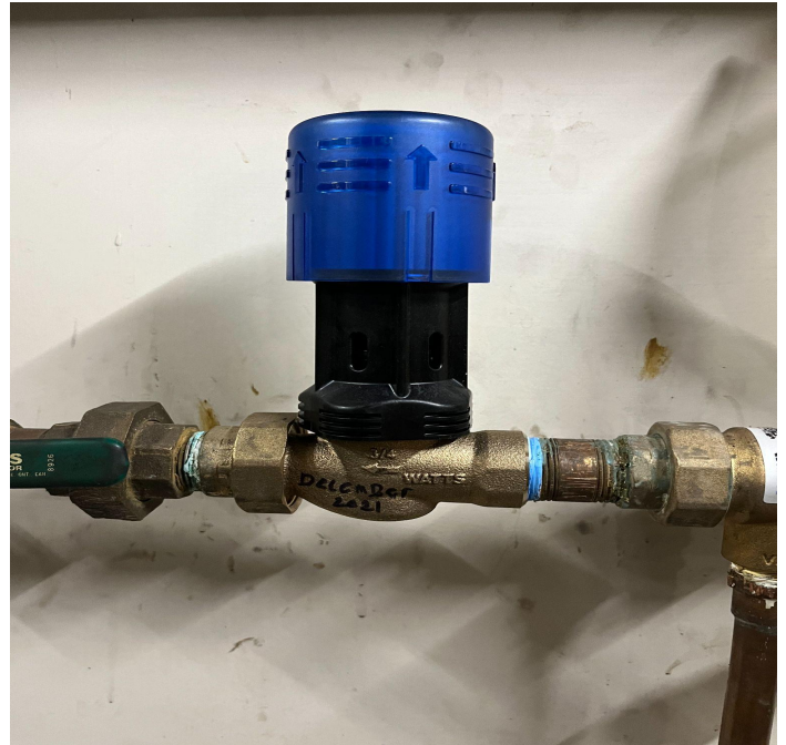
Replaced boiler water feed valve
