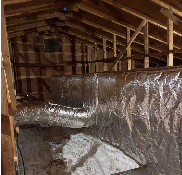
Duct board replacement project
