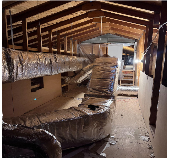
Duct board replacement project
