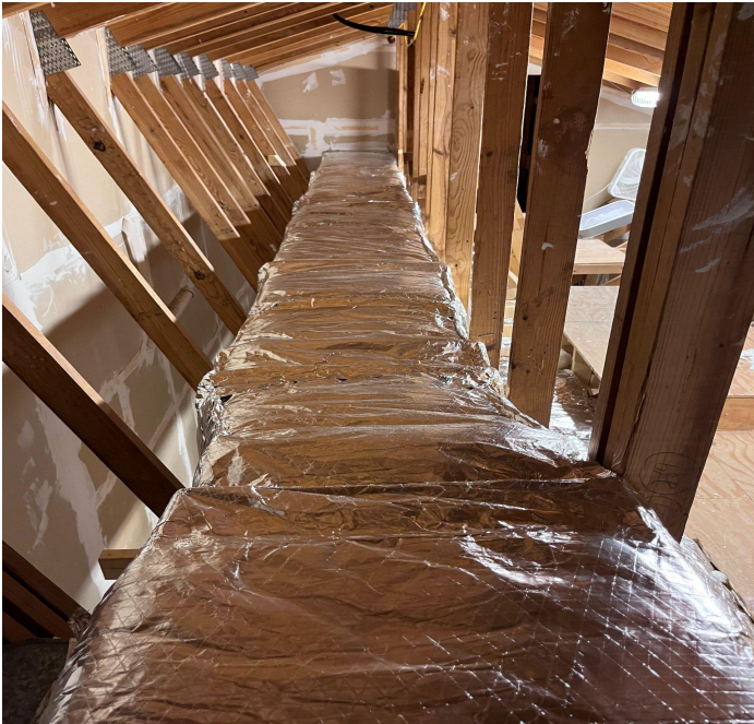
Duct board replacement project
