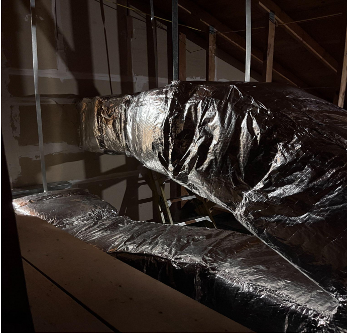
Duct board replacement project
