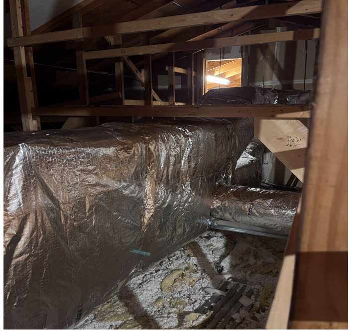
Duct board replacement project
