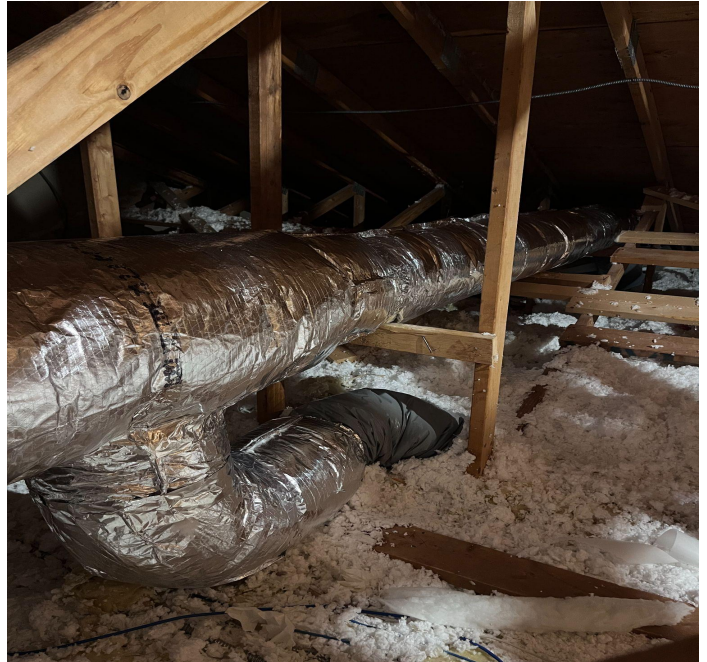
Duct board replacement project
