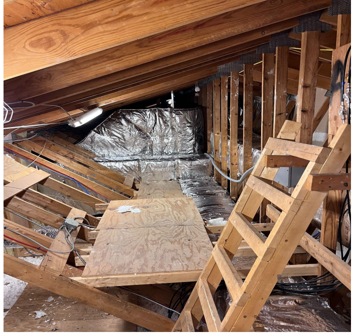
Duct board replacement project
