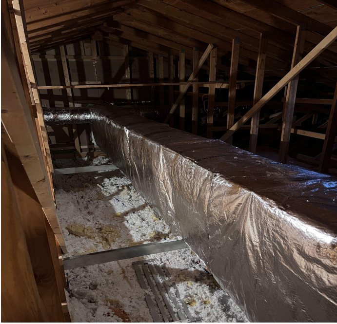
Duct board replacement project
