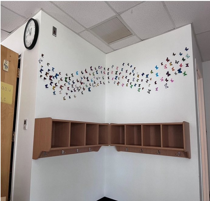
Installation of kindergarten room cubbies
