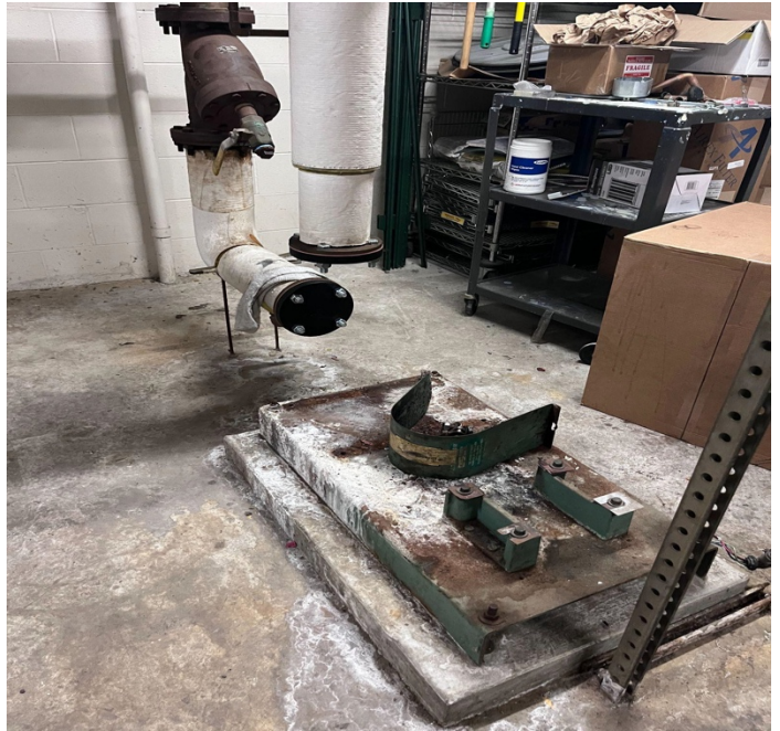
Removal-Rebuild (Right) Taco Circulator pump and motor
