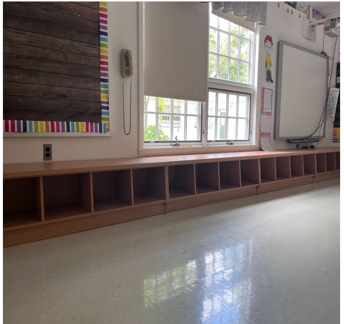
Installation of kindergarten room cubbies
