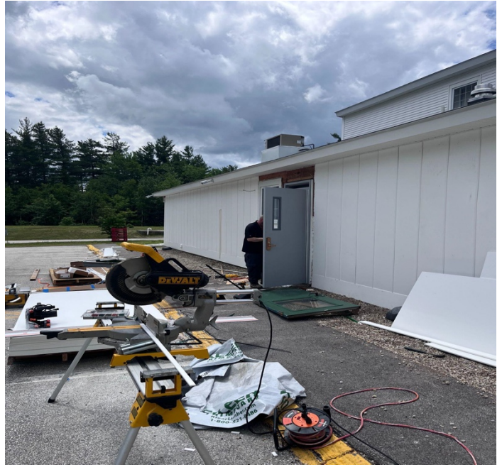
Front siding repairs (in progress)
