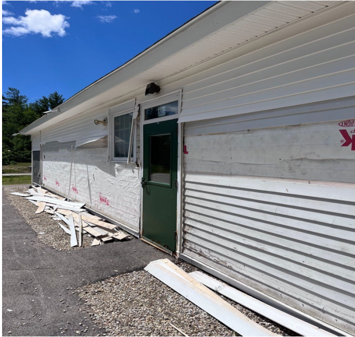
Front siding repairs (before)
