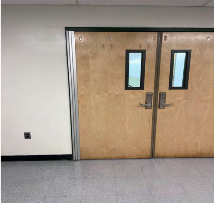
Installed continuous hinge on main foyer hall door
