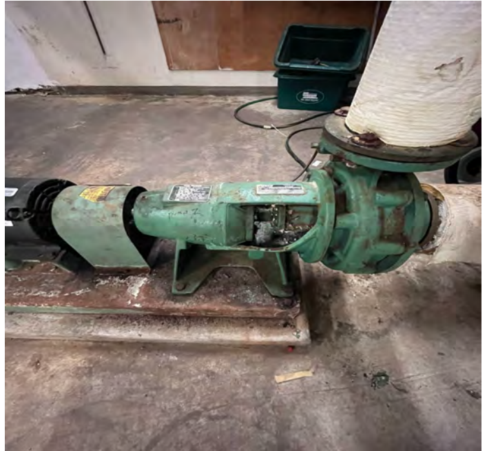
Boiler pump 1 removed for rebuild
