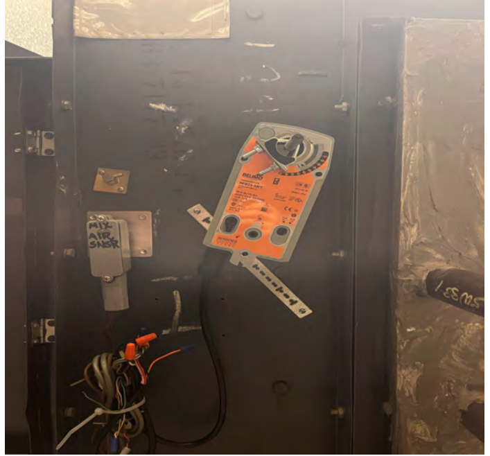
Replaced face & bypass actuator for HV2
