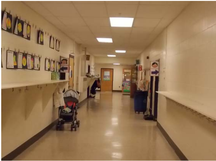
The main hallway has ceiling tiles, painted walls and VCT flooring.
