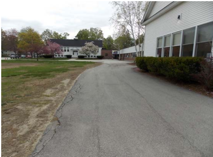
An elevation view with the recent building wing addition in the foreground on the right.
