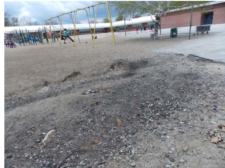
An eroded area at the edge of the playground.
