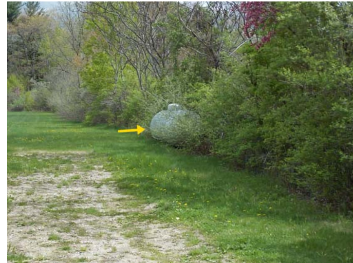
A propane storage tank that is no longer in use.
