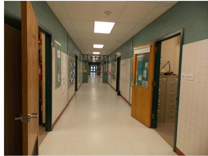
A view of the common hallway.
