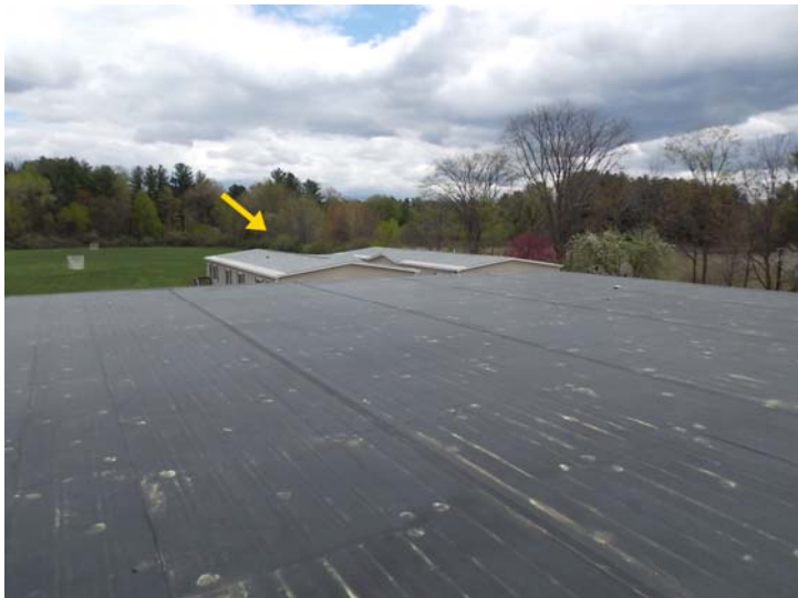
The portable building roofs are covered with architectural shingles.
