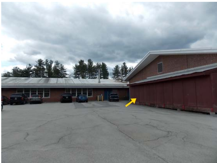
The main building is clad with brick. The storage shed (arrow) is located at the rear of the building.
