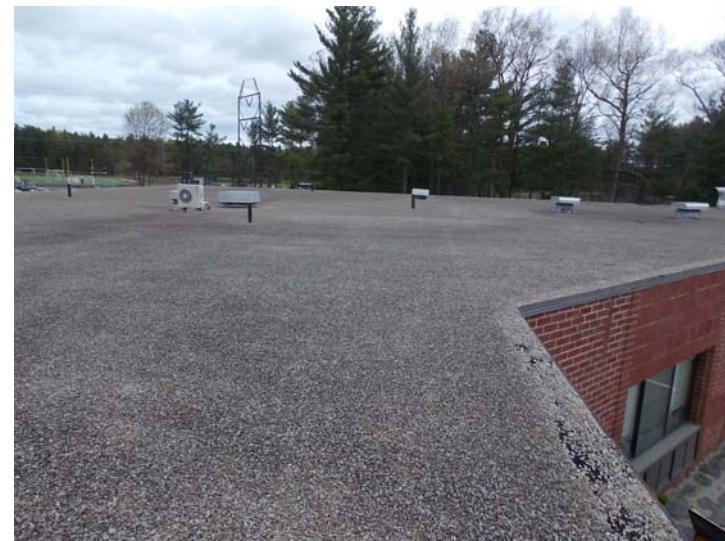
Tar and gravel roof covering on a building section.
