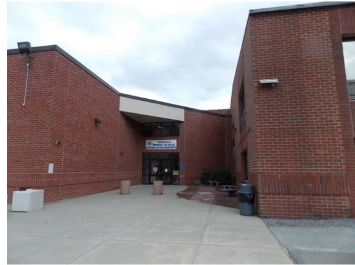
One of the secondary entrances.
