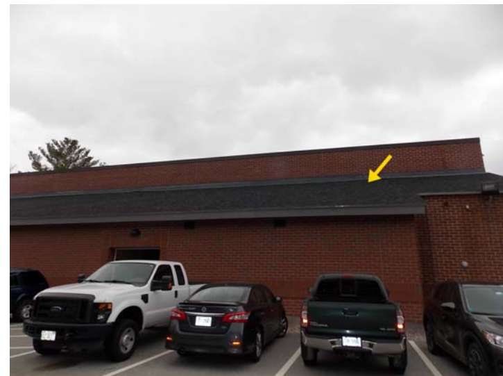
This pitched roof section is covered with architectural shingles.
