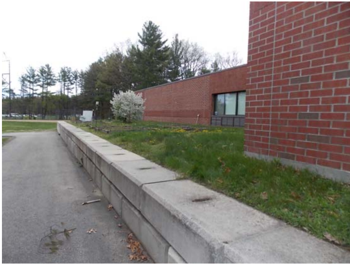
A block retaining wall at the student garden area.
