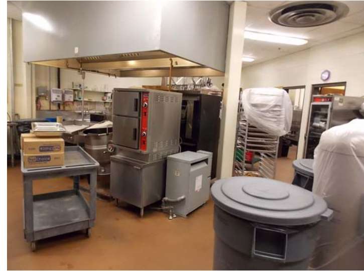
This is the kitchen, which is adjacent to the Cafeteria.
