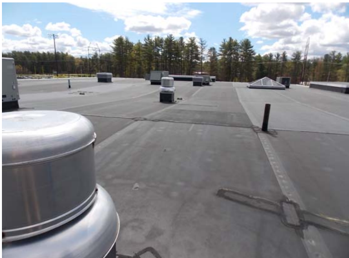
A view of the membrane covering on the annex building's roof.
