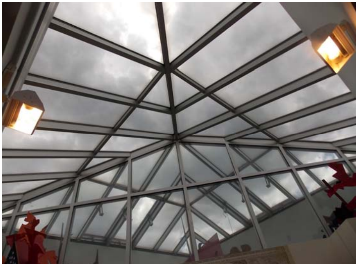
Looking upward at the large skylight in the library.
