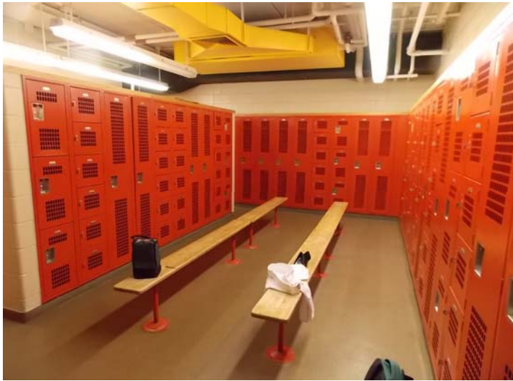
The Girls locker room was found to be in good condition.
