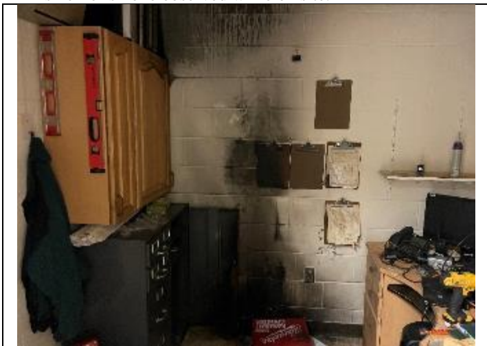
11. View of room 7.
